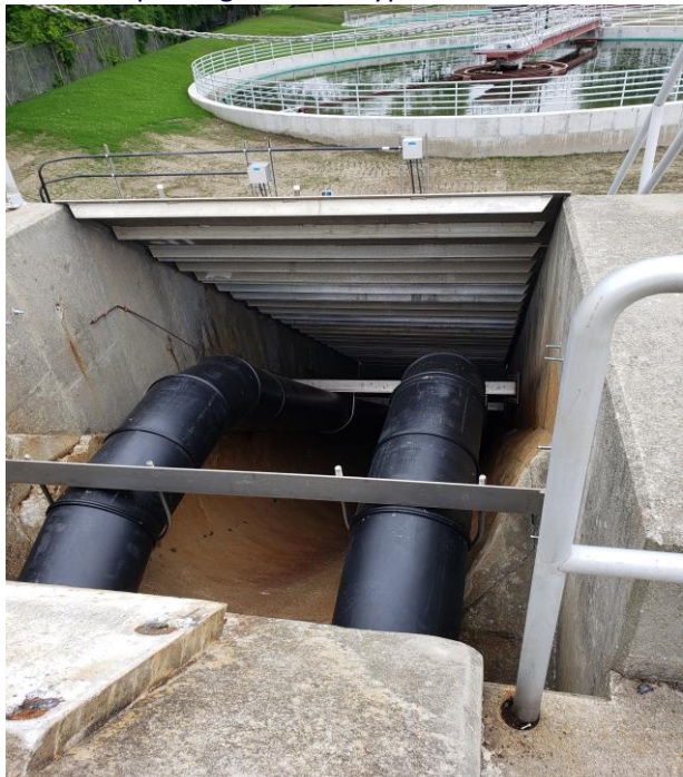
Inspecting Effluent Bypass Conditions
